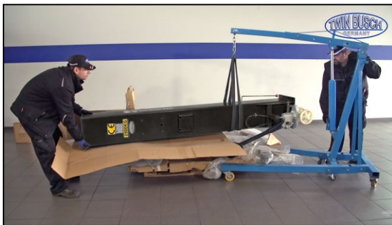
Illustration: Positioning the column
