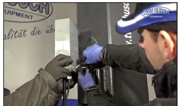
Illustration: Routing the cables through the switch box
