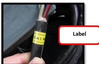
T1, T2, T3 on AC Contactor match with the label on wires.
